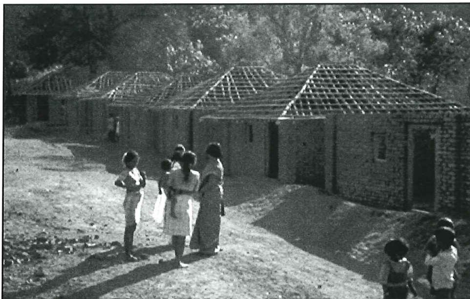
New houses under construction in Shene village. owners.
