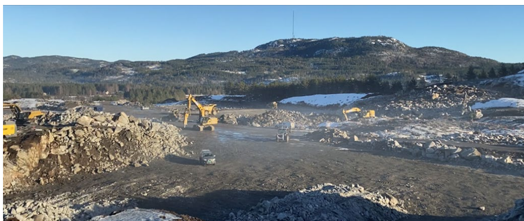
Ongoing site preparation at Åmli, Norway. Photo: Biozin.
