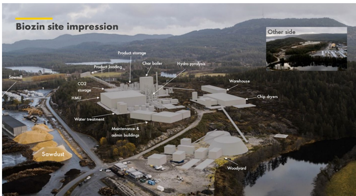
Preliminary 3D-model of the planned Biozin Åmli plant. Photo: Biozin.
