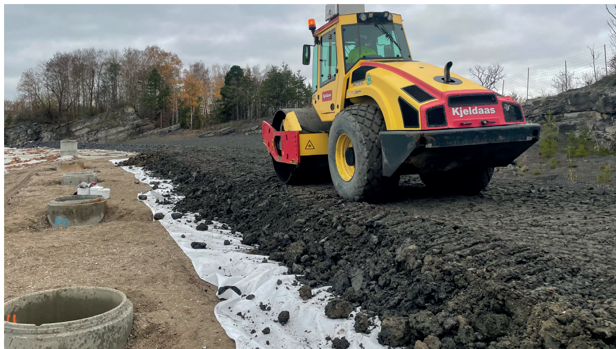
Figure E1: Quantification of large-scale performance under field conditions. Langøya final cover pilot during construction (compaction) of hydraulic barrier and after the application of 1.8-2 m of crushed limestone as frost protection. In addition to measuring the percolation through sections with different waste clays used in the barrier, the sections are heavily instrumented to measure soil temperature, water content and electrical conductivity at various depths.
