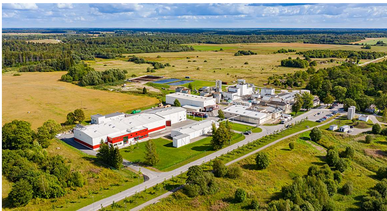
The Lallemand yeast production plant in Salutaguse, Estonia, where the scale-up was conducted.
