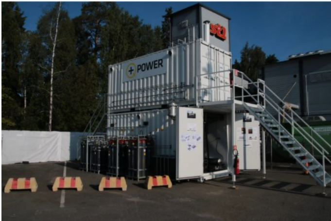
Bioethanol CO 2 sidestream methanation pilot, Vantaa, Finland
